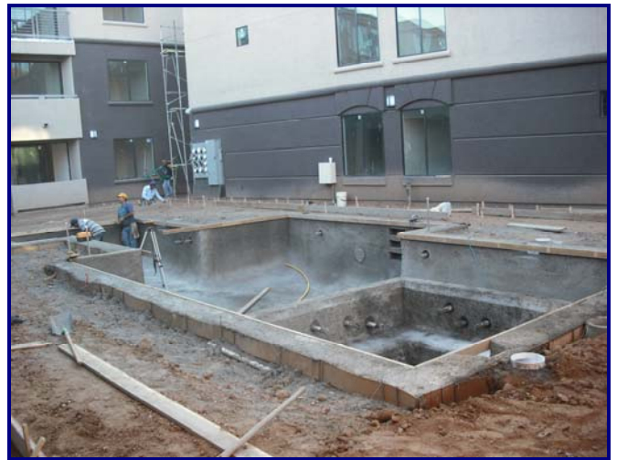
The Clubhouse and pool (above) will be completed 12/12/08.
