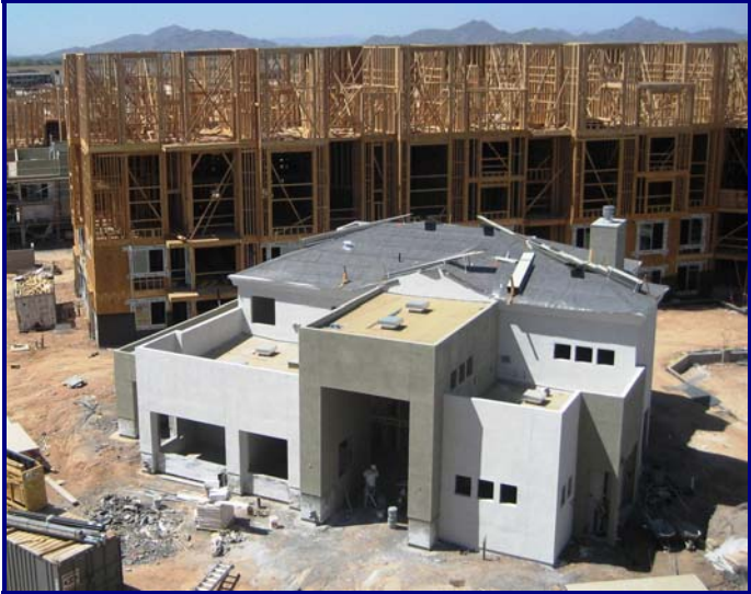
90° PARADISE RIDGE: Clubhouse is 75% complete.
