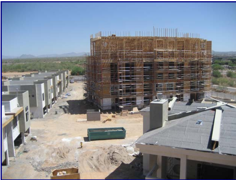
90° PARADISE RIDGE: Building 4 (4 floors) moving along nicely.
